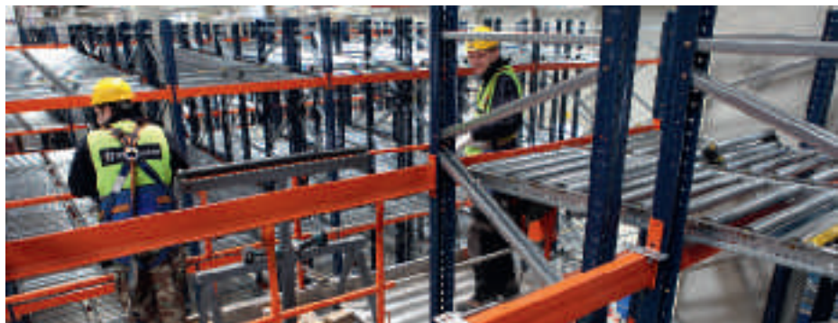
Throughput increased, space used more efficiently: Procter & Gamble replaced drive-in racking with Interroll pallet flow storage at its distribution centre located in Crailsheim (Germany)
