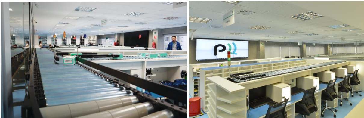
Caption: The Modular Conveyor Platform from Interroll seamlessly integrates into the PLL factory repair service.
